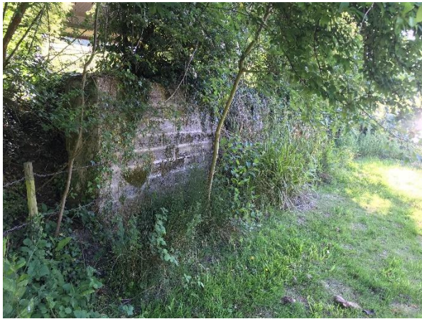
Image 4 – Concrete block retaining wall.
