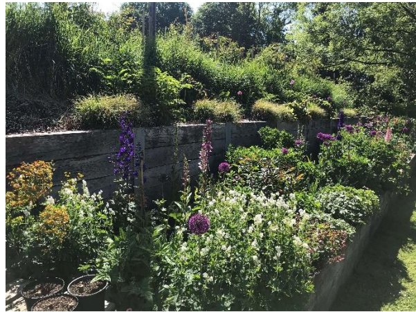
Image 5 – Timber retaining wall.
